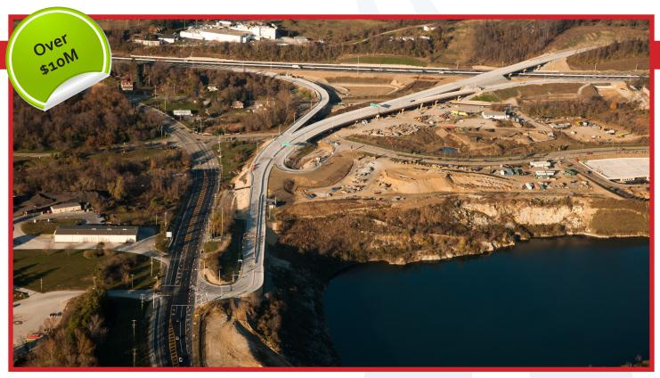
Toll Interchange designated as Interchange 320, where the Turnpike intersected Route 29. The project consisted of adding new eastbound and westbound exit and entrance ramps, mainline widening of the Turnpike to allow for a future six lanes, ramps over the Turnpike, Yellow Springs Road, and Atwater Drive, the construction of three retaining walls, two EZ-Pass electronic tolling facilities and a weigh-in-motion (WIM) monitoring system.
