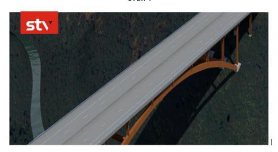
The Hawk Falls Bridge Replacement project will replace aging bridges NB-610 and 611 on the Pennsylvania Turnpike Northeastern Extension (I-476). The existing 738-foot-long structure is functionally obsolete due to lack of shoulders and will be replaced with a new four-lane structure with generous medians and safety shoulders.
